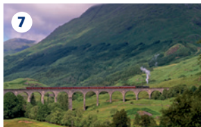
7 THE WEST HIGHLAND RAILWAY – The West Highland Railway's extension from Fort William to Mallaig (opened 1901) saw pioneering use of mass concrete for bridges and viaducts, including the famous Glenfinnan Viaduct. Sometimes described as Britain's most scenic rail journey.
